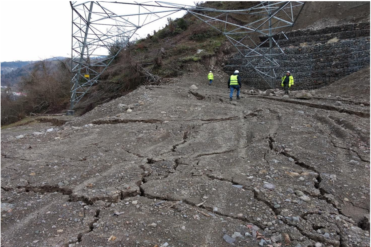
Picture 1: Foundation of Tower # 276
